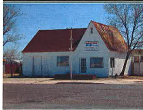
Conoco station (date unknown), Winslow, Arizona. Conforming to Conoco building requirements, this building is characterized by steeply pitched roofs, high, louvered vertical vent, and corbeled eave corners. The building has been modified, with the service garage apparently added later, but is especially notable for retaining its wooden doors in the service bay. Photo: Michael Cassity, 2004.
