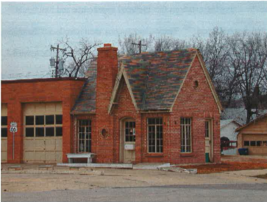
Phillips 66 Station, Chandler, Oklahoma (1930). One of Phillips' many cottage stations, this building conformed to the branded pattern of the company with its Tudor-revival connotations, its chimney, windows, and orange and blue shingles. Note the roundel for the Phillips 66 logo in the chimney and in the right gable. The two service bays at left were added during the period of historic significance as the station added service functions to gasoline sales. Photo: Michael Cassity, 2002.
