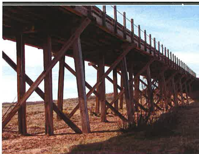
Timber Bridge west of Endee, New Mexico. Photo: Credit, National Park Service, Route 66 Corridor Preservation Program, Santa Fe, New Mexico, 2003.
