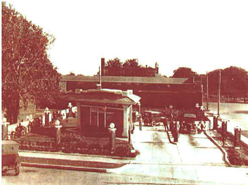
Marland Refining Company Station, El Reno, Oklahoma, about 1925. The Marland stations incorporated a triangular building design that echoed the Marland Oil Company triangular logo. The street in the foreground would become U.S. Highway 66 in 1926. Photo courtesy, Mark Waller, El Reno, Oklahoma.
