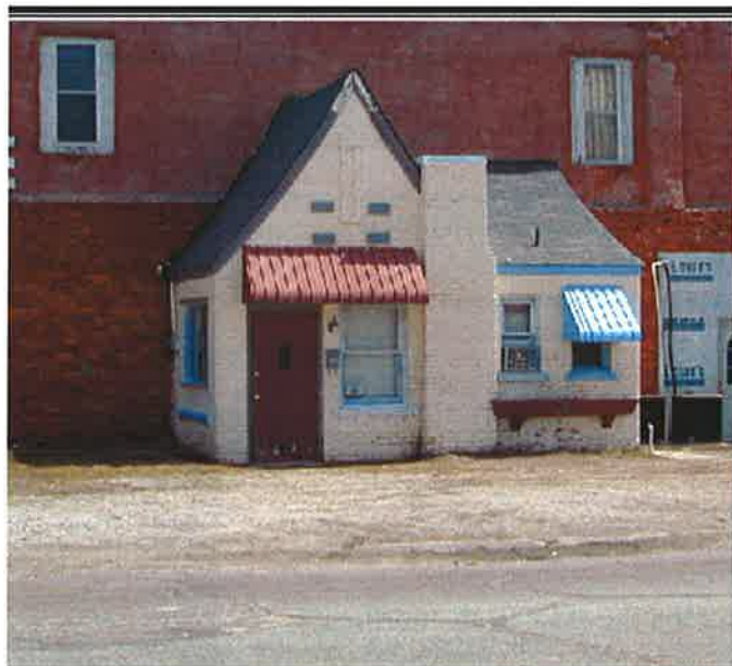
F. D. Mitchell Filling Station (1929 or 1930), located at main intersection in Commerce, Oklahoma, where Highway 66 turned south. Photo: Michael Cassity, 2002.
