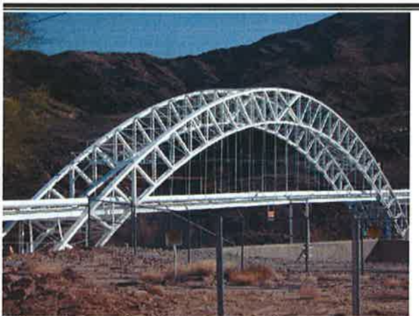
Bridge over the Colorado River at Topock, Arizona (1916), a three hinged steel arch bridge, that served the National Old Trails Road before it became an important Highway 66 bridge. No longer carrying vehicular traffic, its use is restricted to supporting a pipeline. Photo: Michael Cassity, 2004.
