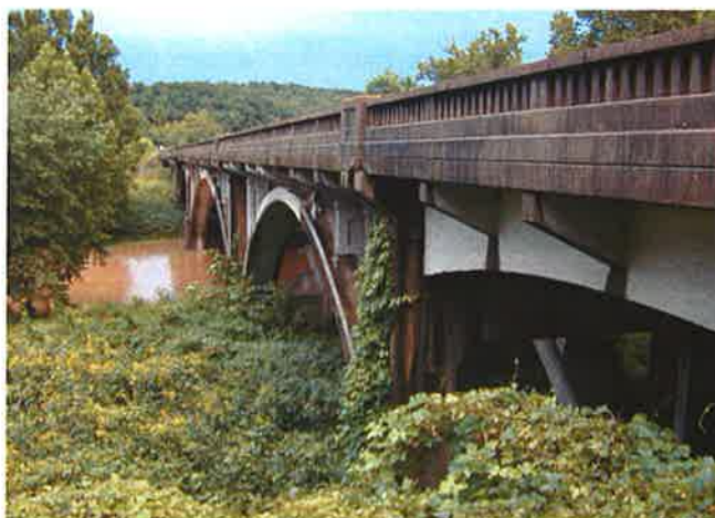
The Big Piney River Bridge (1943) pictured in the post card remains a splendid example of a concrete deck bridge with open spandrel arches. Photo: Michael Cassity, 2004.
