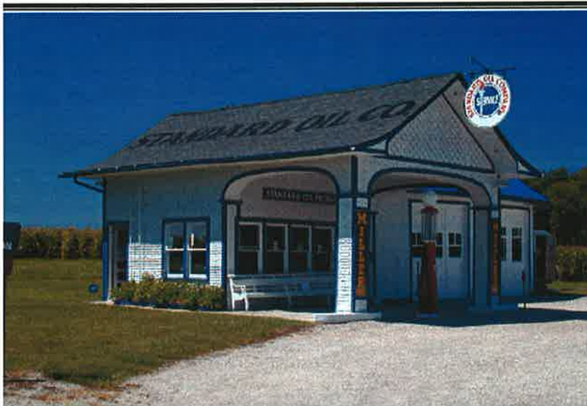
Odell Standard Station, Odell, Illinois (1932). This station, built to Standard Oil Company requirements, has been restored to its original appearance, including, however, the service bays added in 1940. Although the drive has been altered, the original configuration enabled the pumps to be accessed on both sides, with one lane under the canopy and the second outside. A café once was located next to the service station. An example of a house with canopy station, with additional service bays, the evolution of this gasoline station reflects both changing corporate identities (in 1940 it was selling Phillips 66 products and later on it sold Sinclair) and service station functionality. Photo: Michael Cassity, 2004.
