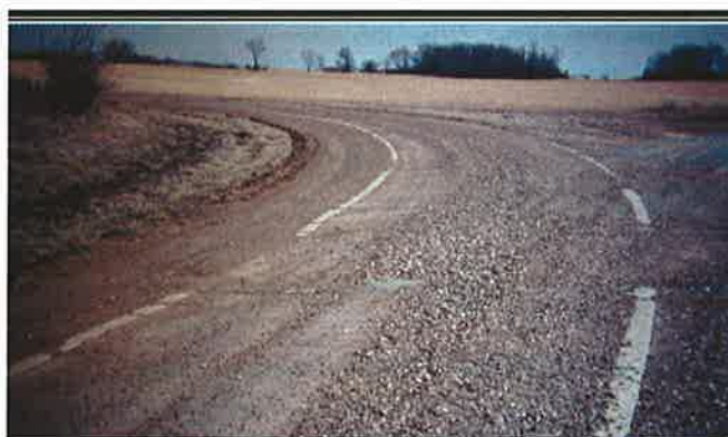
Road turn of U.S. 66 near Miami, Oklahoma where the corner is a 90 degree turn to follow the section lines. This is a section of the highway where the roadbed was only nine feet wide, with concrete curbs on each side. Photo: Michael Cassity, 2002.
