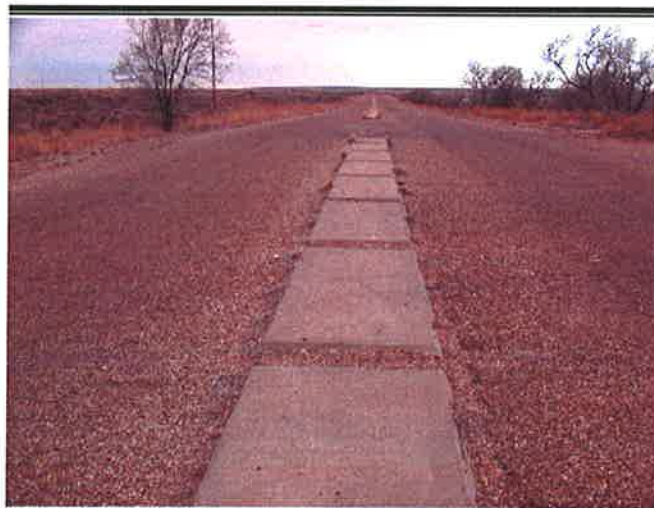
Four-lane Highway 66 looking west into New Mexico, Glenrio. Representative road segment indicating widening of road in towns. Photo: Michael Cassity, 2004.
