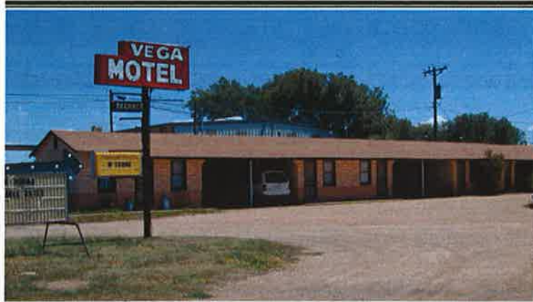
Vega Motel, Vega, Texas (1940). A common pattern was for the motel owner to start with about eight units and later expand by building units in a U-shape with a courtyard in the center, such as at this motel. Photo: Michael Cassity, 2004.
