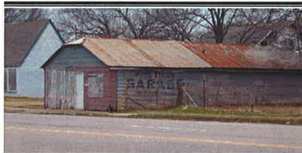
Pike Titus Garage, Stroud, Oklahoma (1931). Although much care went into the creation of this garage (note the clipped gable roof), this, like most small garages, was built to be functional, not pretty. Note the gasoline station adjacent to the left (1925) a common association in the roadside business. Photo: Michael Cassity, 2002.
