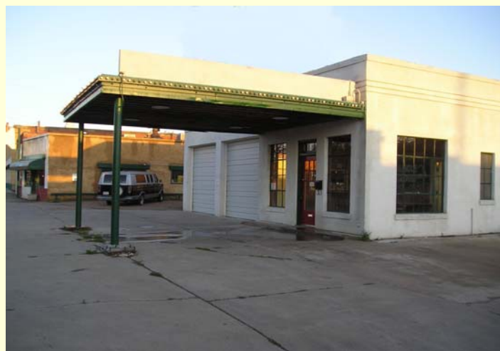
Station canopy, before restoration.
