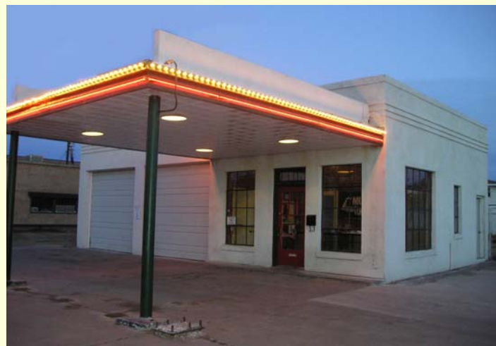
Station canopy, with tin ceiling and lighting restored.
