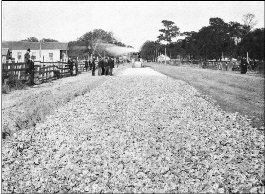
Figure 17. Photograph of an oyster shell object lesson road constructed near Mobile, Alabama ca. 1905, using techniques similar to those used near Beaumont. Source: Project Gutenberg, The Future of Road-making in America , by Archer Butler Hulbert, http://www.gutenberg.org/files/33706/33706-h/33706-h.htm#imagep137 (accessed February 13, 2014).
