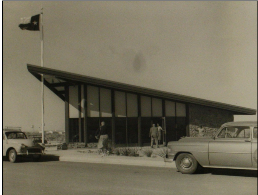
Figure 124. Photograph of a new tourism bureau along the Interstate Highway System, no location, published in the National Highway Week in Texas Publicity Portfolio, May 21–27, 1961. Source: Box 11, Folder 9, Texas Good Road Association Papers, Cushing Library, Texas A&M University, College Station, Texas.
