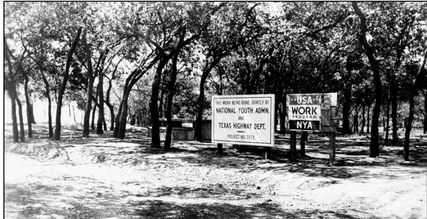
Figure 72. Historic photograph of the first roadside park in Texas, located along SH 71 in Fayette County between Smithville and La Grange. Note signs crediting the work of the National Youth Administration and the Texas Highway Department. Source: Texas Department of Transportation, Media Communications Library, Austin, Texas.
