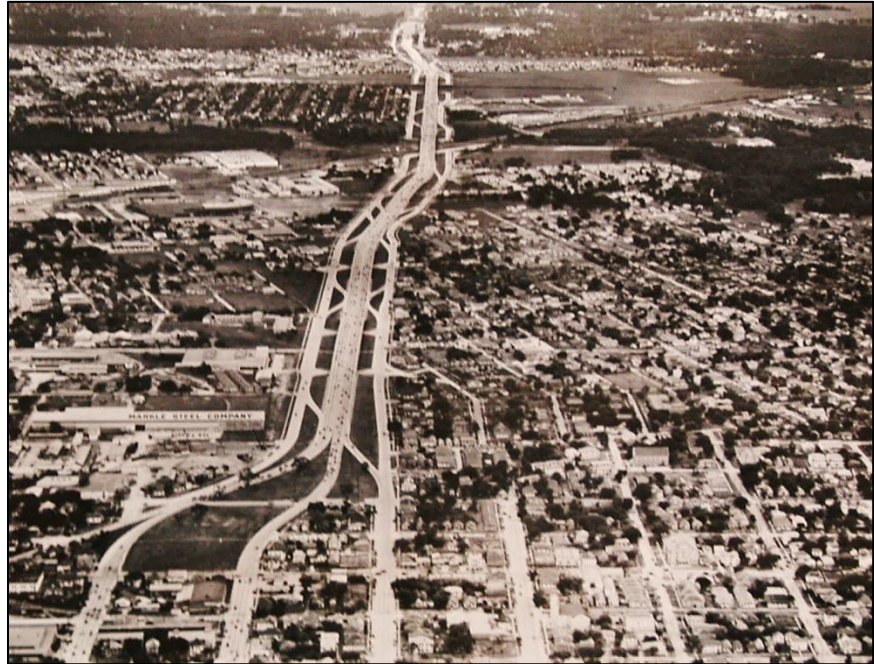
Figure 106. Photograph captioned, "The new Gulf Freeway through Houston, Texas, July 1949. The parallel side roads serve local traffic movements." Source: Photo no. 49-1926, Box 107, Record Group 30, Photograph Collection, National Archives, College Park, Maryland.
