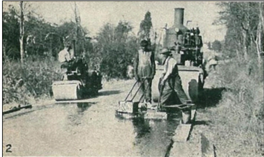
Figure 18. Photograph showing workers applying a seal coat to an object lesson road ca. 1905, illustrating the labor-intensive process of road construction. Source: "Back in Time: The Object Lesson Road" by Rickie Longfellow, FHWA, https://www.fhwa.dot.gov/infrastructure/back0607.cfm (accessed February 13, 2014).
