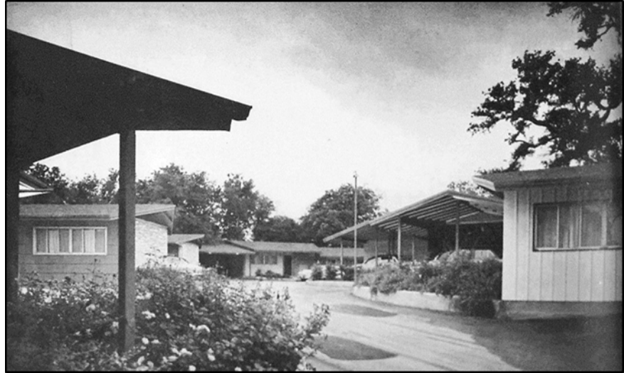
Figure 112. Photograph of the Terrace Motor Hotel in Austin, featured in Architectural Record , vol. 114, no. 1 (July 1953), page 172. Note the sprawling layout of the building, the surface parking lot, and the integrated carports adjacent to each unit. Source: Architecture and Planning Library, University of Texas, Austin, Texas.
