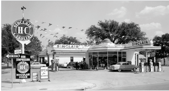
Figure 7-29. The above Sinclair gas station, once located in Austin, is an example of the corner lot design with a circular central office and two canopies.
