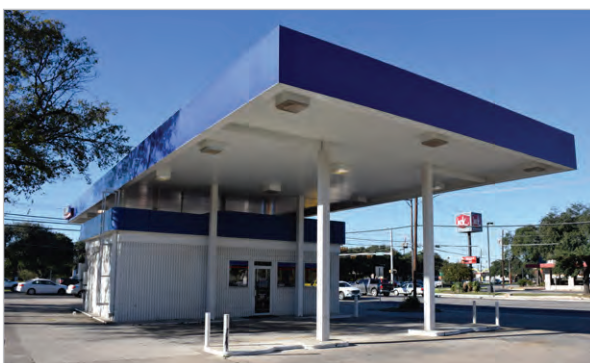
Figure 8-3. After 1970, oil companies typically constructed high, well-lit canopies over pumping areas. This configuration allowed all types of vehicles access to pumps while protecting customers from the weather.
