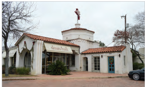
Figure 12-17. The original canopy of this former Magnolia station, located at 5424 Austin Highway in San Antonio, was enclosed with glass. Note that the glass is set back within the canopy, so that the original canopy features are still recognizable. This station falls within the Tier 2 integrity assessment category and has significance under Criterion A for its association with the Meridian Highway and under Criterion C for its quality of design. Since the glass enclosure of the canopy is sympathetic to the building's overall design, the alteration only minimally affects the building's integrity. Other alterations, including removal of original signage and gas pumps, are minimal.
