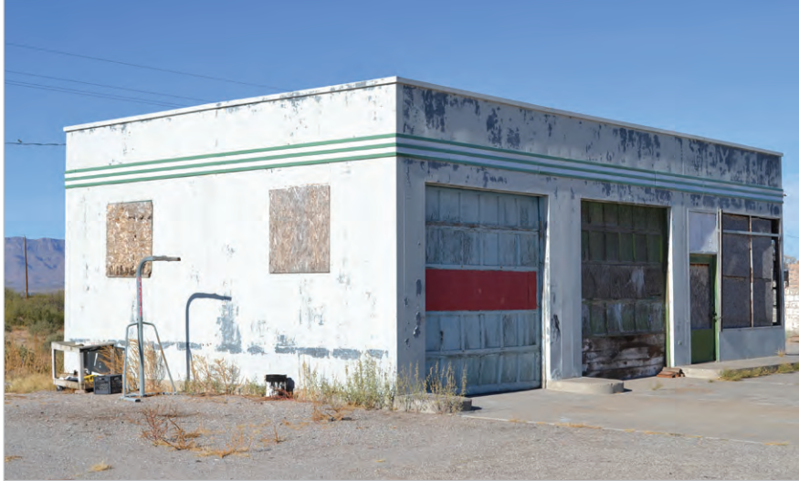
Figure 12-5. This c. 1940 Texaco station on SH 20 in the vicinity of McNary is individually eligible under Criterion C: Architecture as a good and intact example of Walter Teague's design of the Type A gas station for the Texas Company, a once prevalent and common form that is becoming increasingly rare in Texas. The form remains unaltered, but loss of design elements includes stars and signage. In addition, the loss of the window panes and overall deterioration of the building affects integrity of materials. Despite this, the fenestration pattern remains intact and the building's loss of integrity is minimal.
