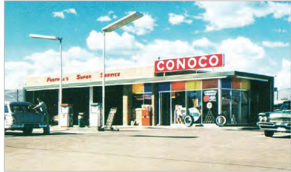
Figure 7-8. This is an example of a 1960 Conoco station without a canopy. Conoco would often use brightly colored panels in the transoms to grab the driver's attention.
