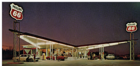
Figure 7-22. This 1960s Phillips 66 station (location unknown) features a projecting triangular canopy and large slanted plate glass display windows; known as the “batwing” design.
