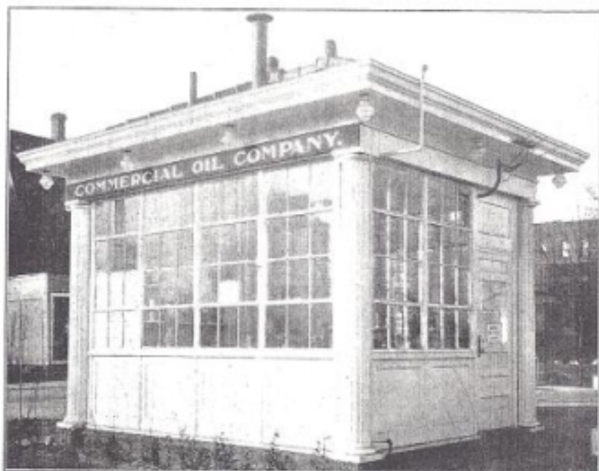
A four column type of Union Metal filling station installed by The Commercial Oil Company, Cleveland—a particularly practical station for limited space.
