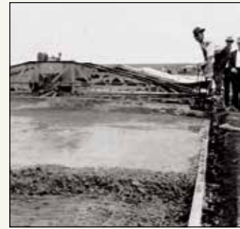
Left: Placing and pouring concrete on the Bankhead Highway; Texas Federal Aid Project No. 45 (Tarrant County). Middle left: J. P. Punk McNatt Motor Co. Olds-Cadillac in Greenville (Hunt County).
