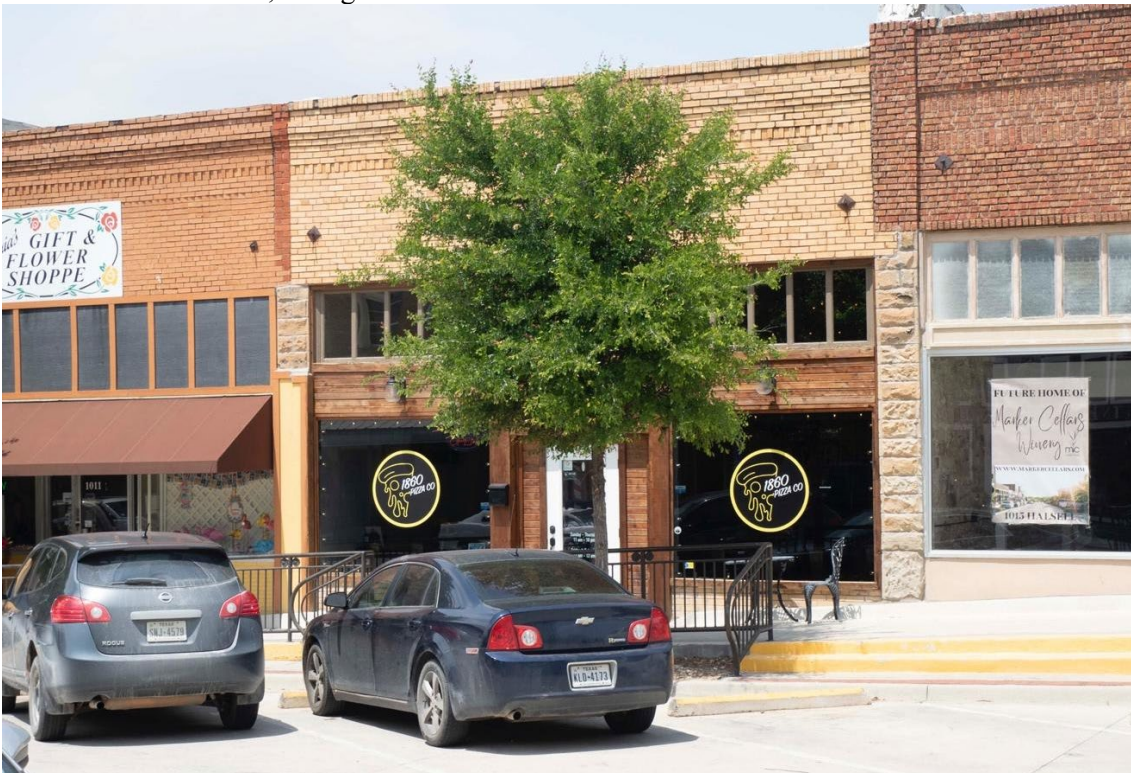
Photo 22. Resource 24, facing northwest.
